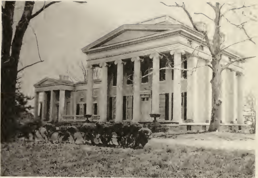
Figure 45. Fatland Ford as rebuilt for Dr. William Wetherill sometimes attributed to the design of John Haviland. (Reproduced from Faris, Old Roads Out of Philadelphia , 1917.)
